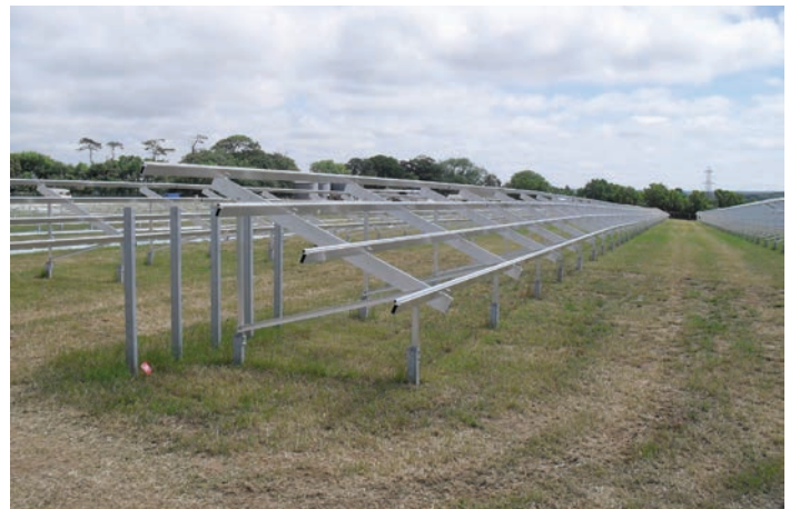
Figure 14 The ground anchors and framework associated with the development of the 1.4MW Benbole solar farm in Cornwall.
