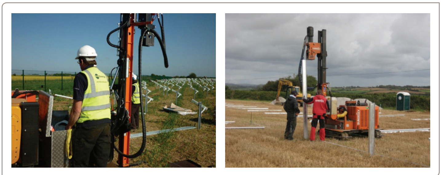
Figure 16 Where pile driven foundations are proposed consideration should be given to the noise impact at nearby sensitive receptors. Difficult ground conditions, such as those encountered at the 1.4MW Wheal Jane solar farm shown here, may also require drilling.
