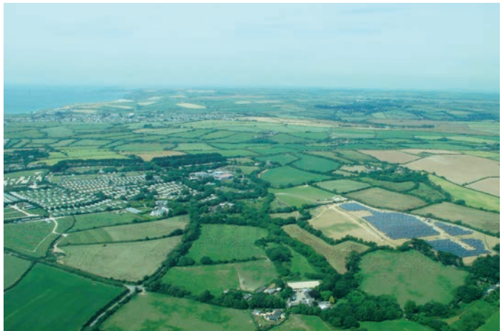
Figure 3 The development of a 1.4MW solar farm on land adjacent to the Hendra Holiday Park, Newquay will greatly assist in meeting the electricity demand of this facility. Images courtesy of Hendra Holiday Park.
