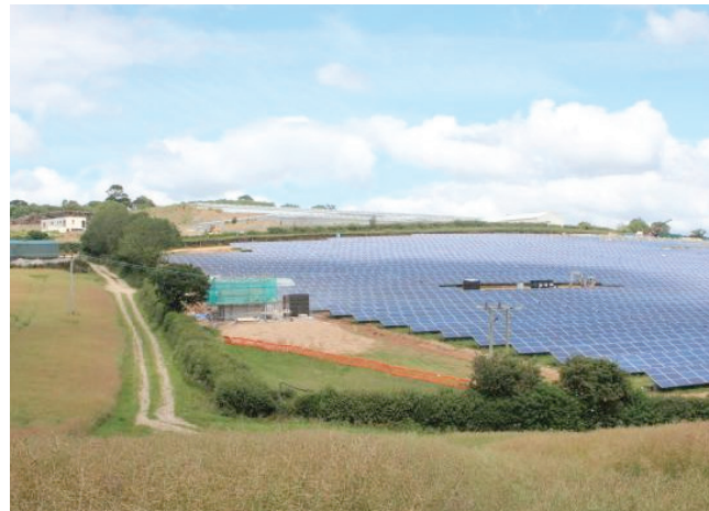
Figure 17 The 5MW Howton solar farm in Cornwall. Image courtesy of Lightsource Limited.
