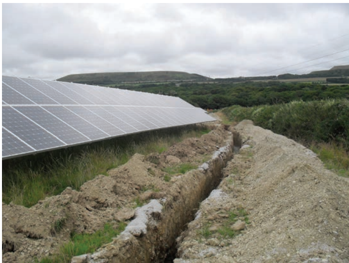
Figure 9 Soil excavation during cable trenching at the 5MW Trefullock solar farm in Cornwall. Note how topsoil and subsoil are stored on opposite sides of the cable trench in order to avoid the mixing of soil types and facilitate subsequent soil replacement and site restoration.
