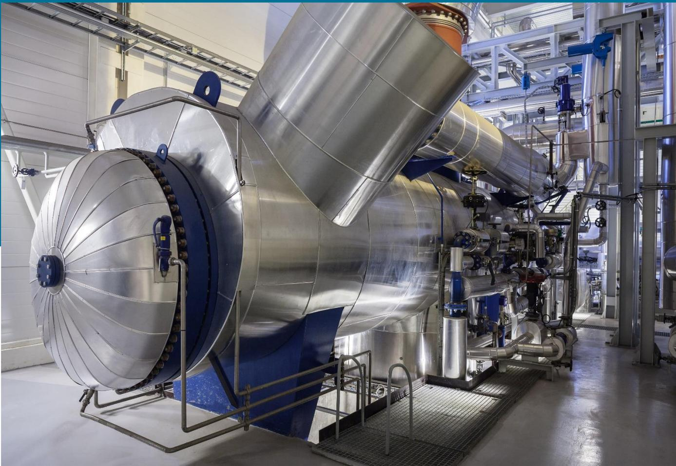
Cover photo: Steam turbine condenser of a cogeneration plant. Image sourced from IStock.
