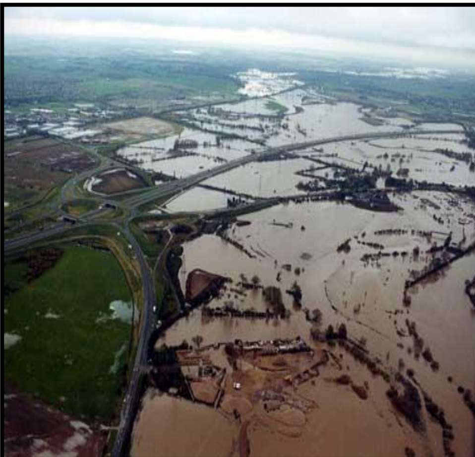
Understanding ground conditions is critical to flood resilience. Here extensive and vital infrastructure has been put out of action by flooding
