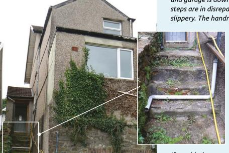
To make matters worse, the rain-water drainage discharges directly onto the steps which means that they are always wet. Following a very cold night they would have ice on them. As this is a regularly used accessway this is deemed to be a Category 1 hazard to a vulnerable elderly person.
