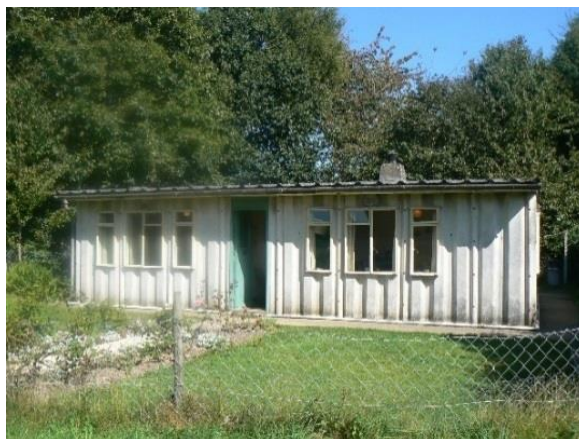
Photo: In 1945, 40,000 Arcon 'prefab' council bungalows were built from a steel frame clad with asbestos
