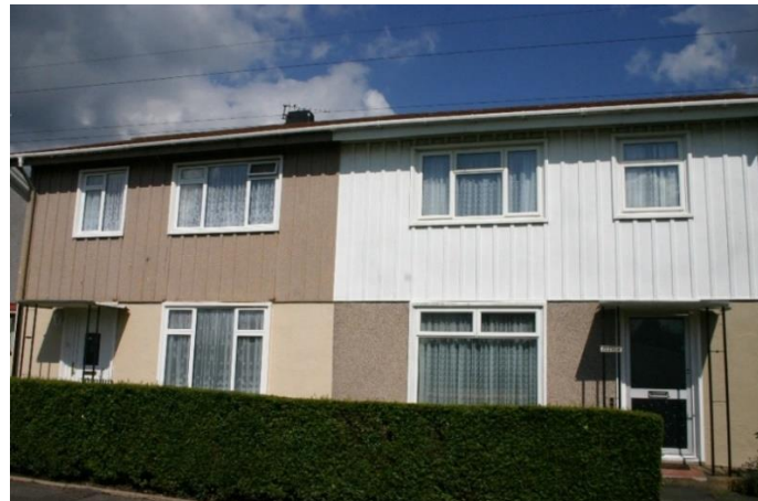
Photo right: 'BISF' steel frame and cladding system, of which 35,000 were built between 1945-1950. Photos below: Local children playing outside their steel framed homes (1960s)
