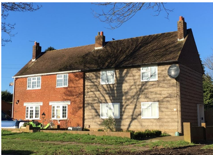
Photo: A pair of 'Airey' houses built with pre-cast concrete systems, which are designated 'defective'. The RTB semi on the left has had the structure replaced by traditional cavity brickwork, while the semi on the right has been repaired by the council but retains the original design.
