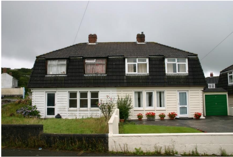
Left photo: 'Cornish' concrete frame/panel system, of which 30,000 were built between 1946-1960
