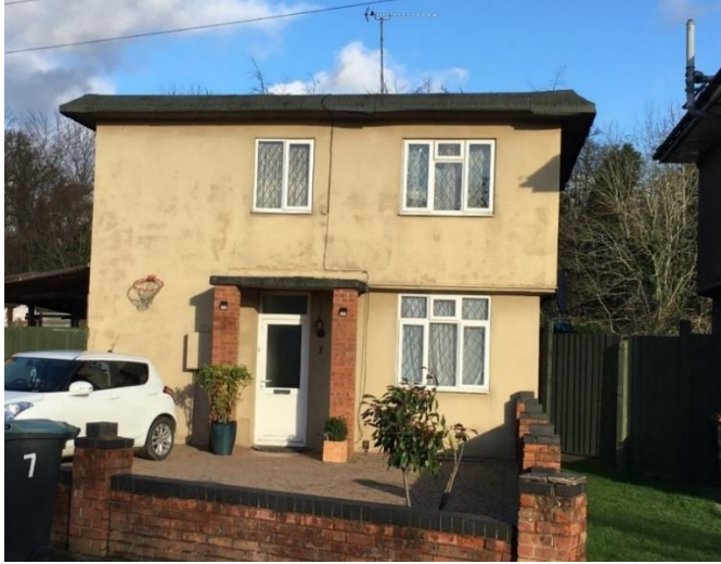
Left photo: Experimental in-situ concrete frame house, built by BRS, Hertfordshire 1946 (as it appears in 2020)
