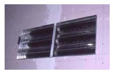
Plate 8. Multi-blade damper mounted in Dry-lined partition
