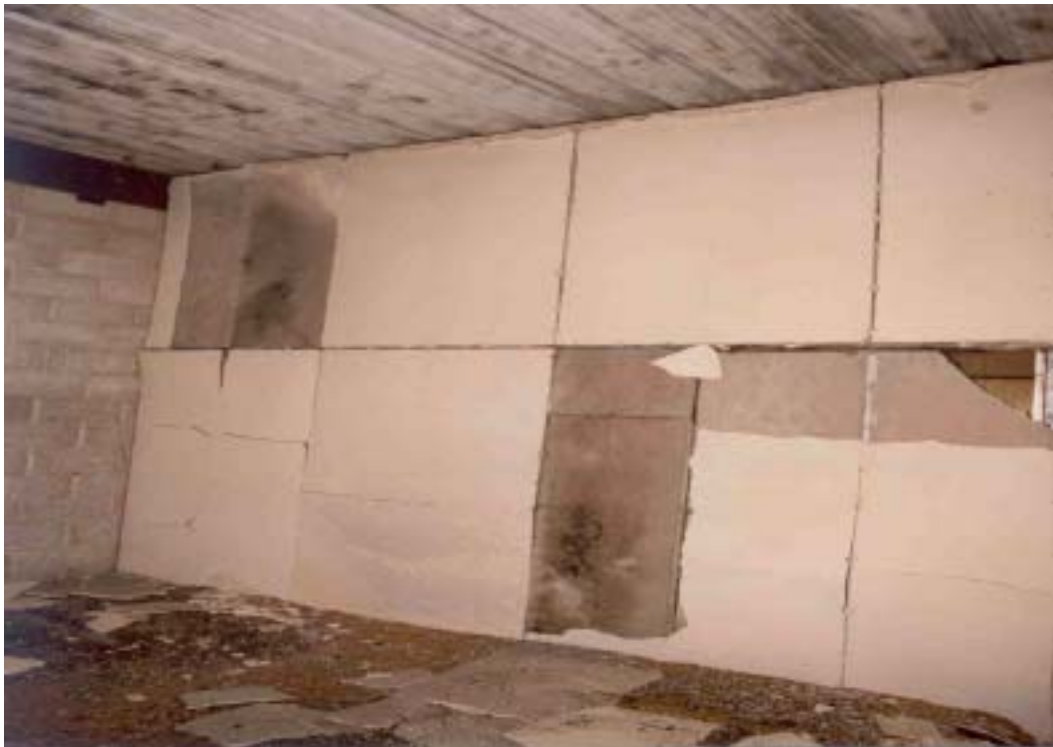
Figure B12 BRE corner compartment – interior view post-test
