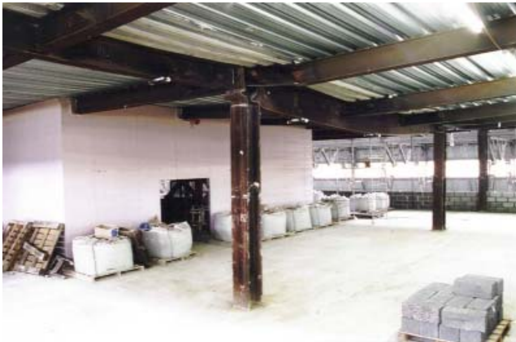
Figure B7 Plane frame – post test (note: localised buckling at top of column)
