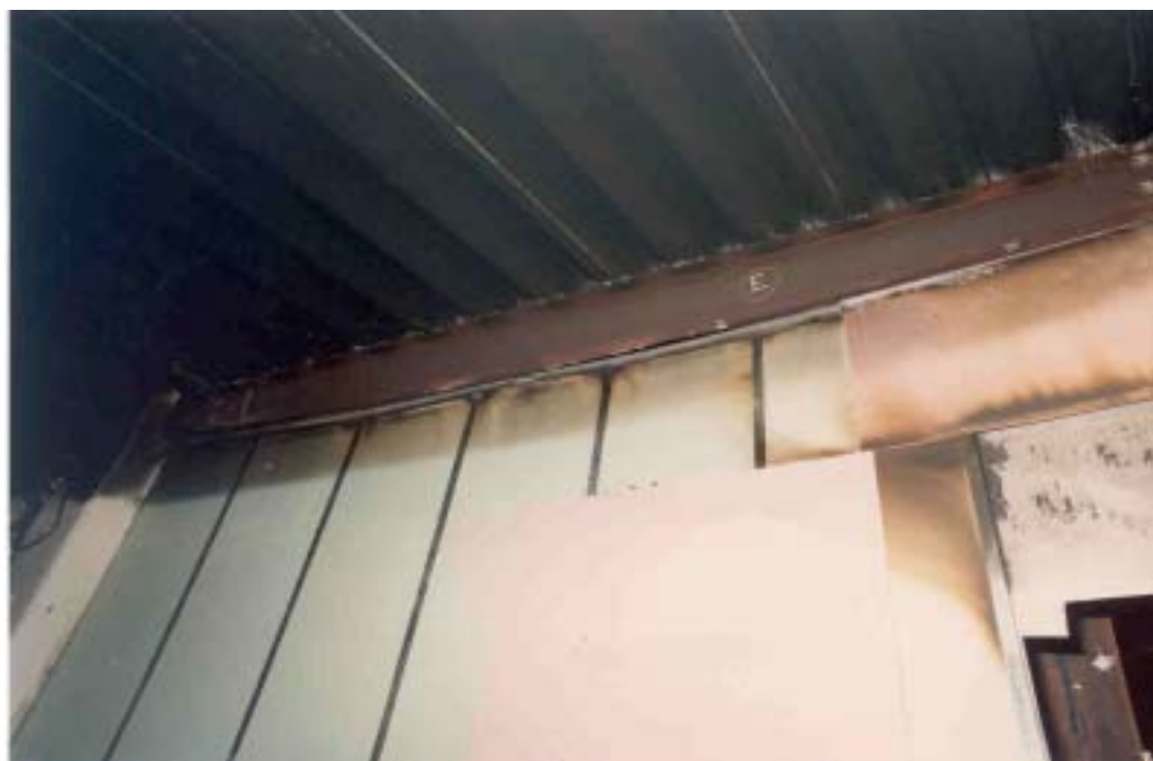
Figure B13 BRE corner fire test – exterior view post-test
