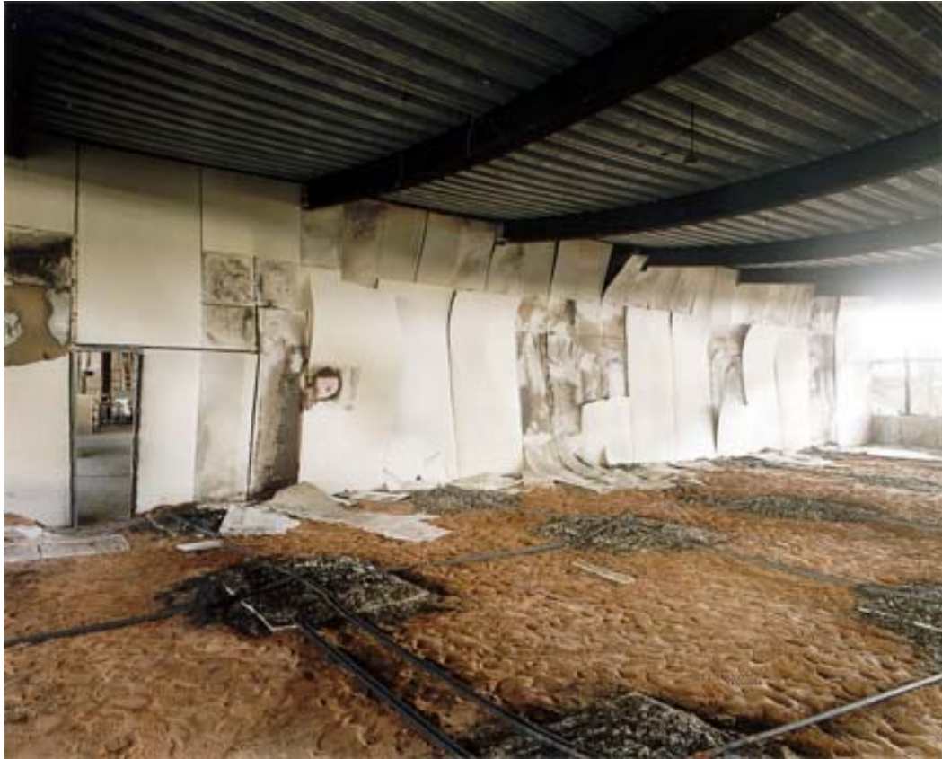
Figure B19 Deformation of floor slab causing instability of compartment wall – BRE large compartment fire test
