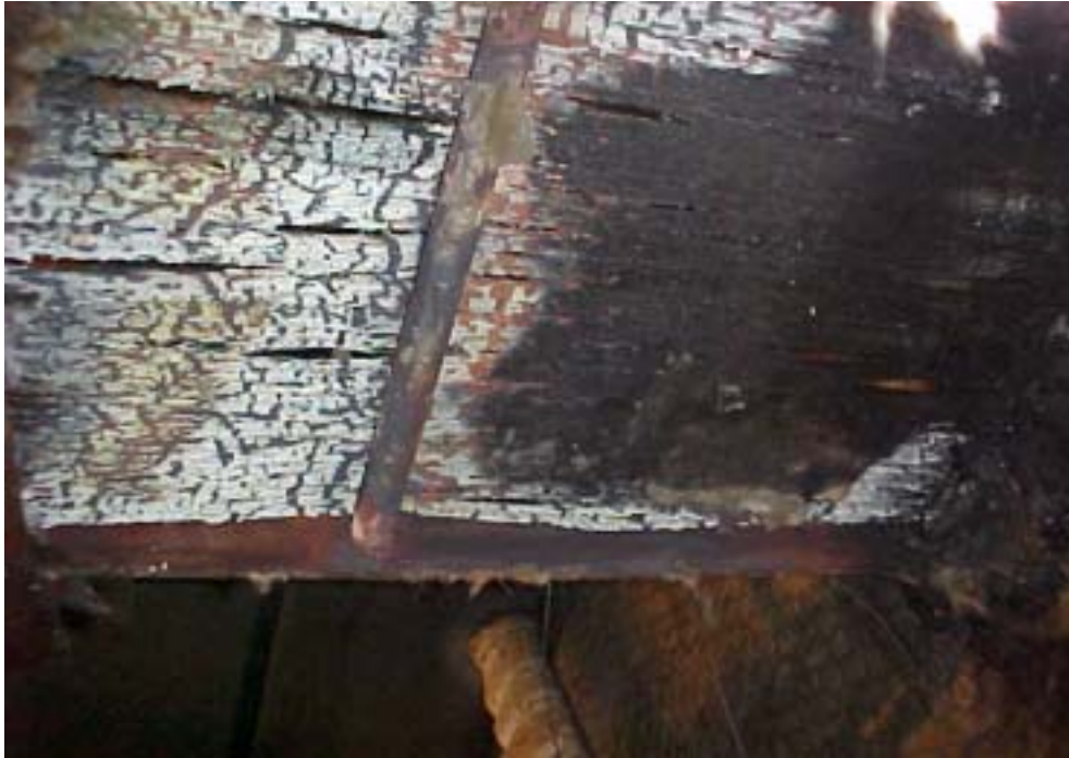
Photograph B9. Post test in the ceiling void with a cavity barrier.
