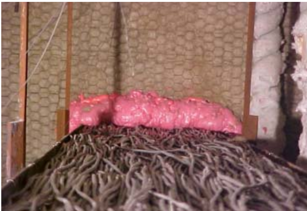
Photograph B6. Fire stopping in the cable ladder adjacent to the cavity barrier.
