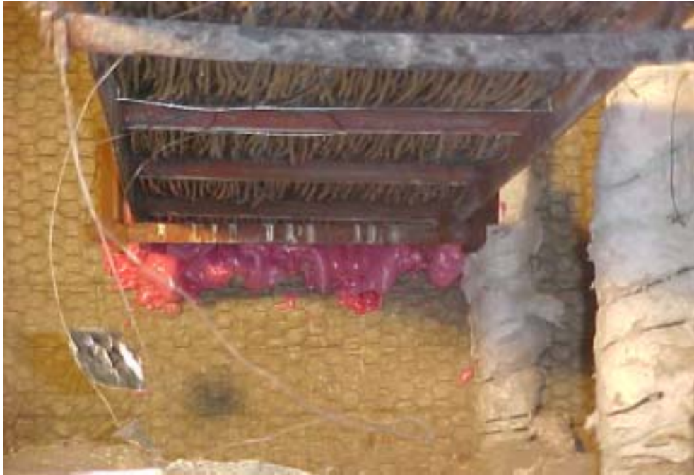
Photograph B7. Fire stopping to the underside of the cable ladder adjacent to the cavity barrier
