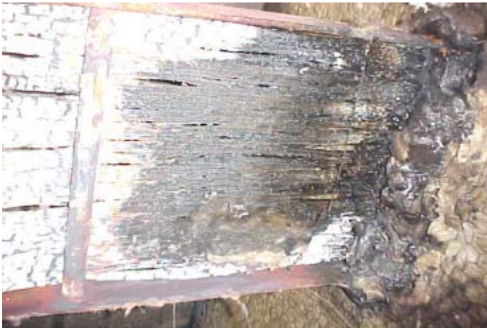
Photograph B10. Cavity barrier with fire stopping around the cable ladder.
