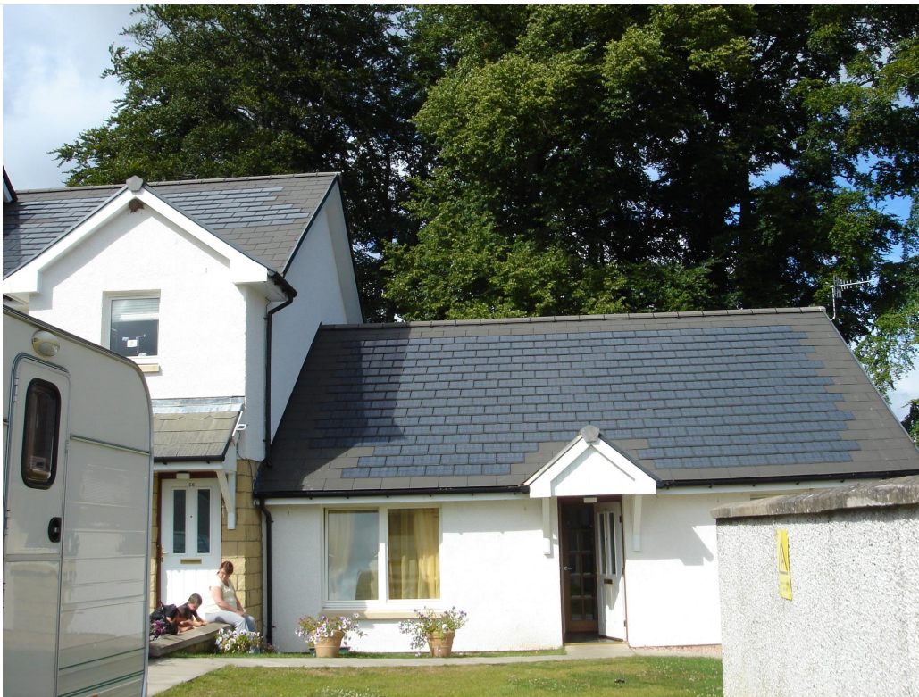
Figure 63: Roof-integrated array with crystalline silicon roof tiles, where the left-hand side of the array is shaded by the adjoining building. At the extreme left of the picture some shading of the upper roof array can be seen.
