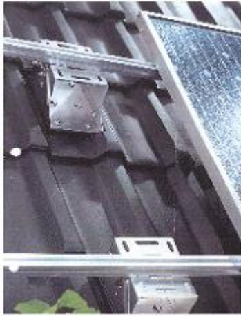
Figure 24: Klover Tile with Special Attachment (picture Klover)
