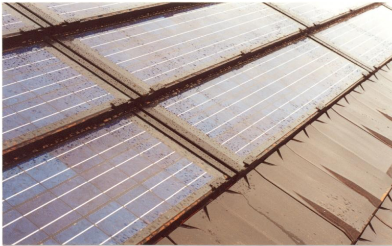
Figure 6: The complete Pfleiderer module (Solar Century)
