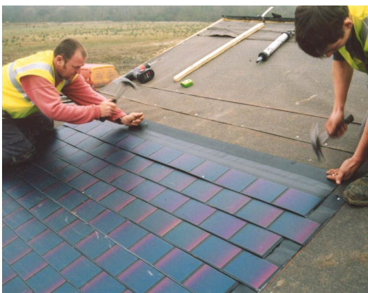
Figure 13: Shingle installation on felted board
