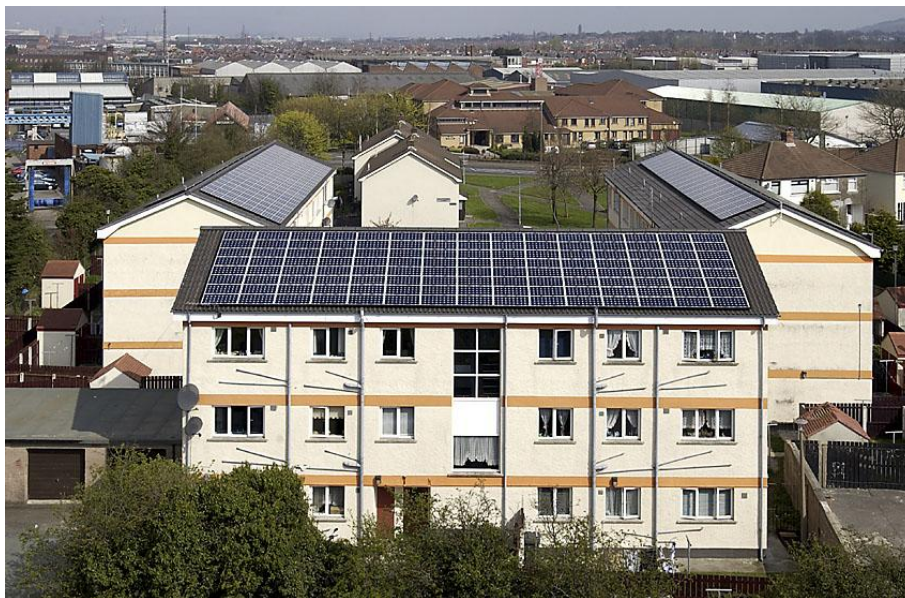
Figure 21: “Sun-in-a-box” system: laminates landscape, base structural rails vertical
