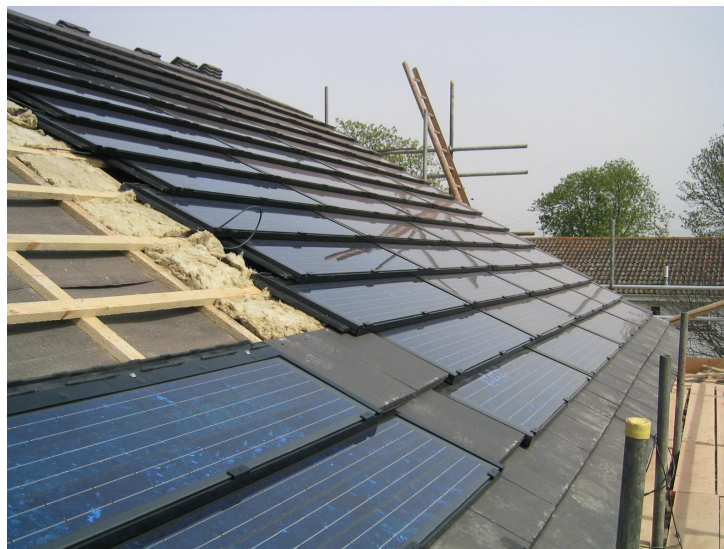
Figure 7: Installation of the Pfleiderer Terra-Piatta solar roof tiles (BRE)
