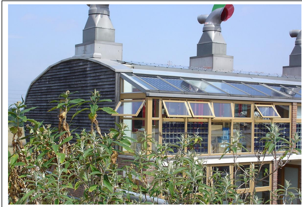
Figure 34: The modules mounted on the roof and wall of the conservatories
