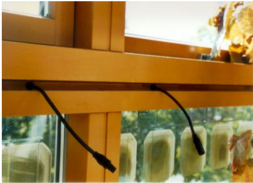
Figure 35: Once plugged together, the plug and socket connectors will be concealed and accessible
