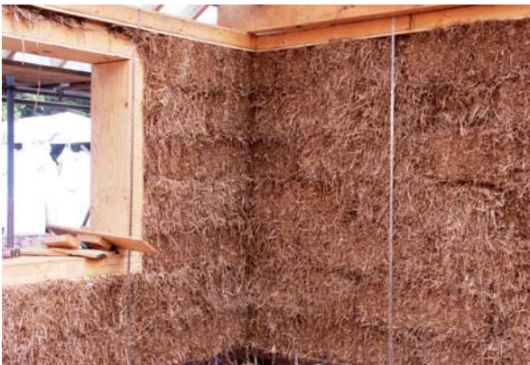
Figure 8: A completed wall with straps connecting the wall plate to the base (Courtesy of Mike Beckett/Collins & Beckett)
