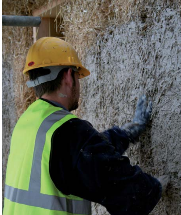
Figure 9: Vapour-permeable render being applied to exterior of straw bale surface (Courtesy of Mike Beckett/Collins & Beckett)
