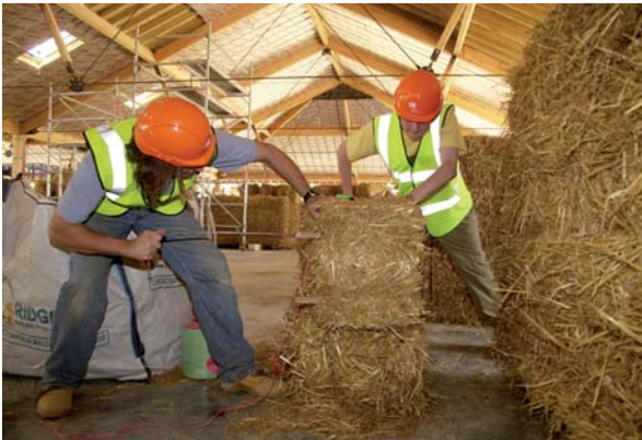
Figure 7: Pinning, tying and cutting end bales (Courtesy of Mike Beckett/Collins & Beckett)
