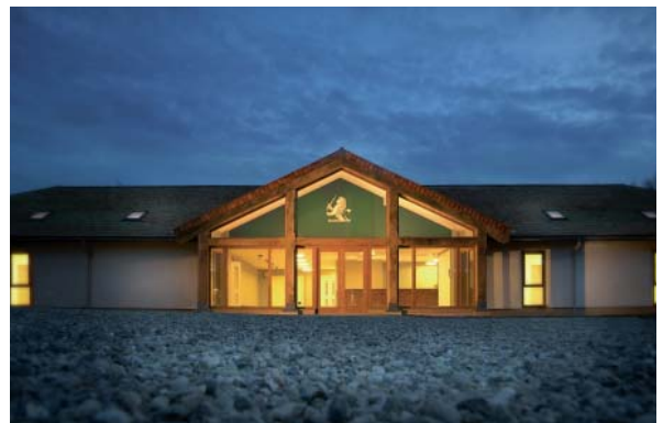
Figure 1: Sworders' auction rooms, Stansted Mountfitchet, Essex – a single-storey 1100 m 2 building, constructed in 2008 using straw bale wall construction (Courtesy of Mike Beckett/Collins & Beckett)
