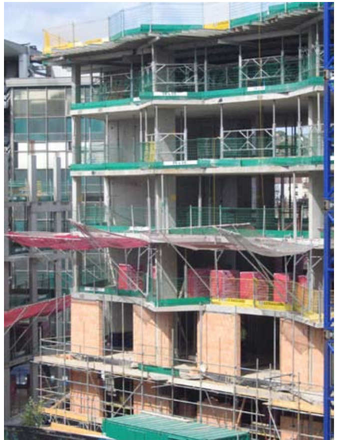
Blockwork going in between concrete super-structure (NBT)
