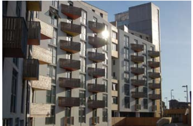
Newly completed (NBT)
