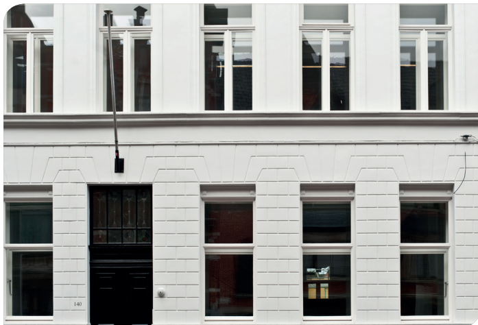
Oude Houtlei 140 in Ghent, headquarters building for Bopro, a sustainably refurbished listed building assessed to BREEAM In-Use, BREEAM In-Use award winner 2011
