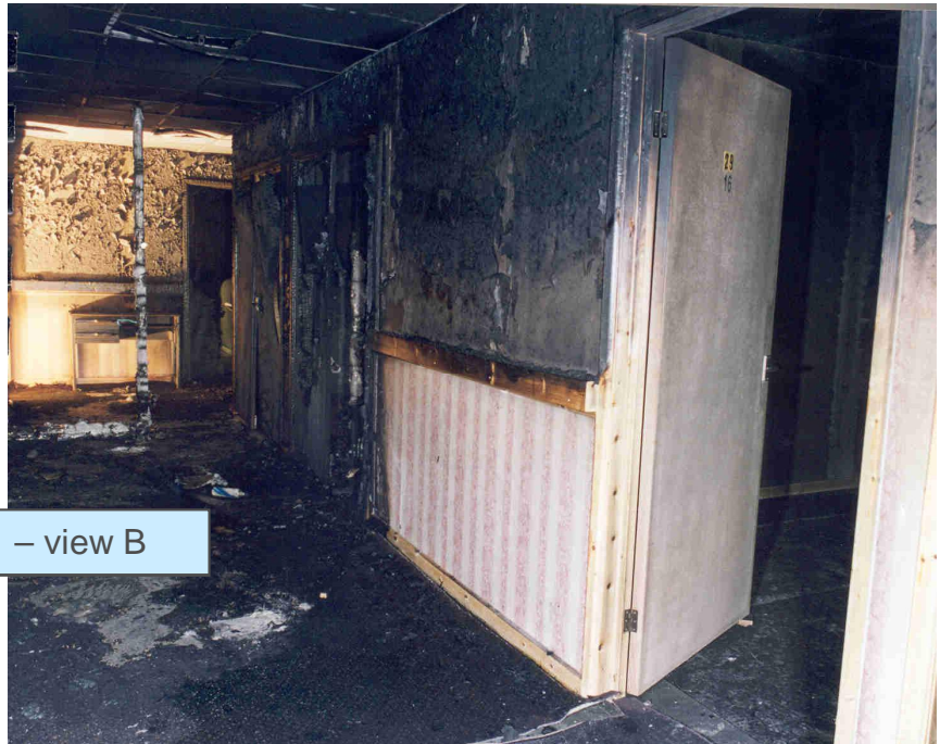
Before Test 1 – view B
