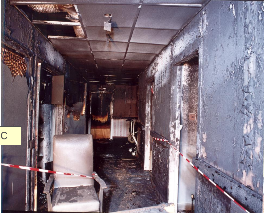
Lower Ground Floor – view C
